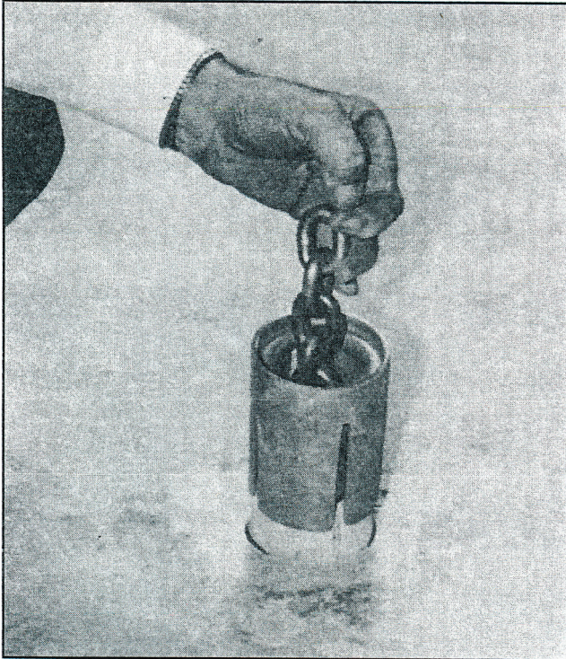
Insert assembly anchor into hole as shown. Use both hands if necessary.
