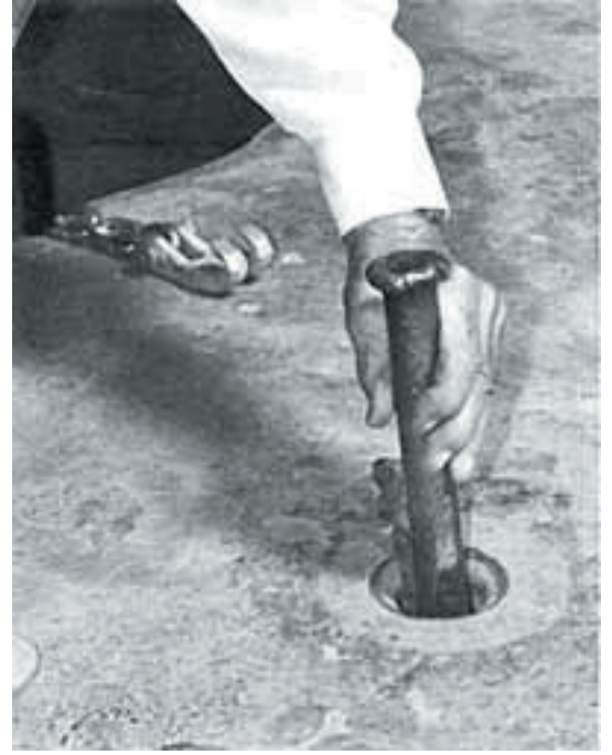
Position driver on edge of anchor expander on the opposite side of the chain retaining wedge.
