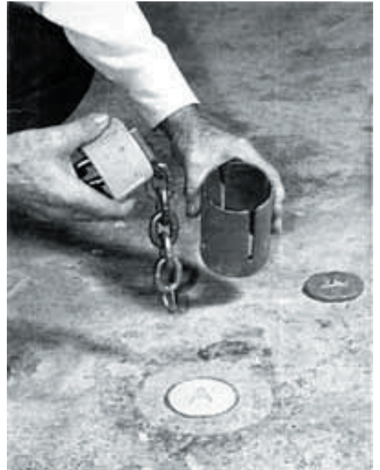
Grasp anchor sleeve and pre-assembled expander and chain.
