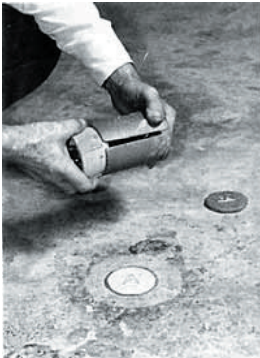
Firmly insert anchor expander with chain into anchor sleeve.
