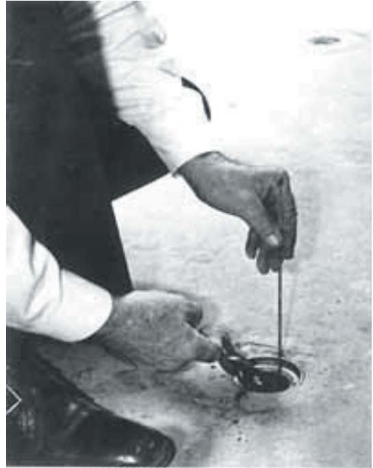
Insert hooked end into slot at top of chain retaining wedge.
