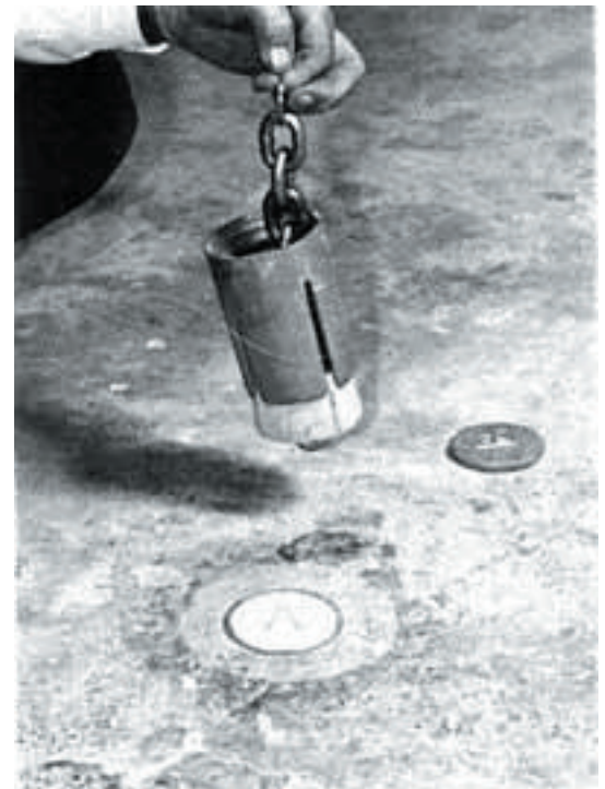
Hold assembly by wire ring making sure anchor expander is evenly aligned to sleeve.
