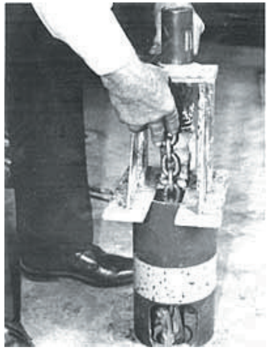
Attach chain to puller claw removing all the slack.
