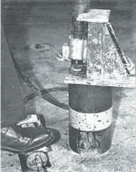
Slowly apply pressure to pump. Sleeve should easily rise from hole in floor.
