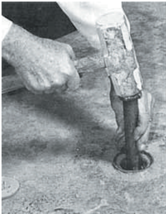
Striking a firm hammer blow, dislodge anchor expander from anchor sleeve. Take care not to damage retaining wedge.
