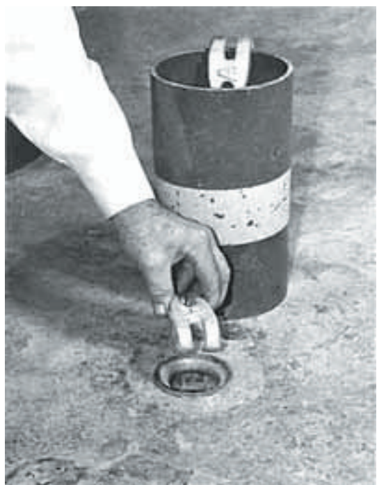
With anchor expander dislodged from anchor sleeve, attach puller claw to protective ring at top of sleeve.
